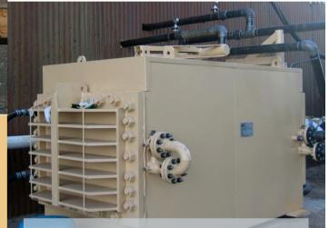
Water and Direct SLUDGE-to-SLUDGE Heat Recovery
