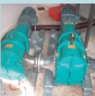
**In plastic recycling** there is a simultaneous demand of washing and macerating. The Multicrusher / Rotary Lobe Pump package ensures reliable particle size reduction and reliable plastic / water transfer.
