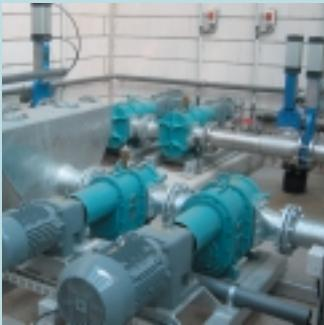
**In Waste Water Treatment Plants**, rags and stringy materials are often a problem for pumps, valves, instruments and controls and other downstream equipment. The Multicrusher with „Pull-In Function“ macerates and reduces these troublemakers to unproblematic sizes.
