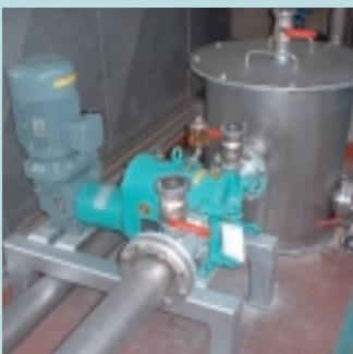
**Raw Sewage** often is loaded with rags and textile products. The Boerger Multicrusher takes care of these foreign objects to prevent blockage downstream. The pictured unit is compact and allows Ease of Maintenance through the Quick Release Cover.
