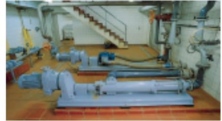
Fig 1: Comparison PC/Rotary Lobe
